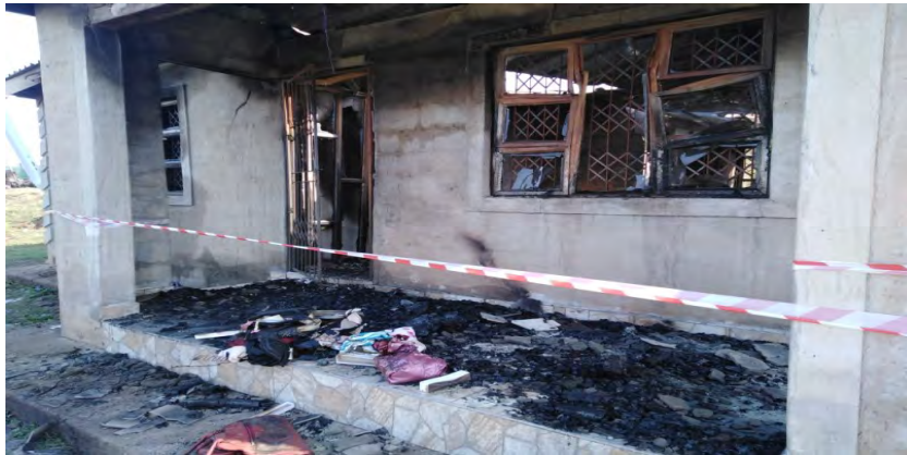
Figure : Conveys the aftermath following the structural fire incident that resulted in one fatality in August 2020 in Ward 26, Ntshawini area.
