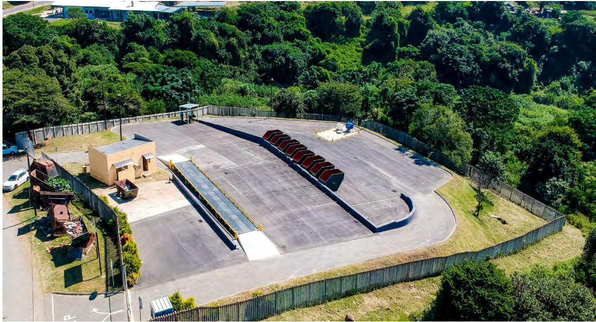
Waste Management Section - Completed KwaDukuza Waste Transfer Station
