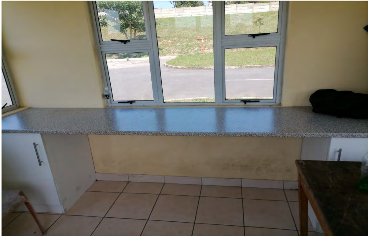
Refurbished guard house with new cupboards and countertop
