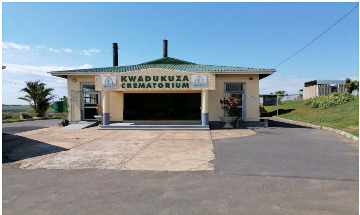
Cemeteries and Crematoria Section - Revamped KwaDukuza Crematorium - new aluminum doors
