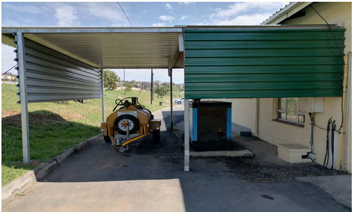
Extended shelter for the backup generator and the diesel tank
