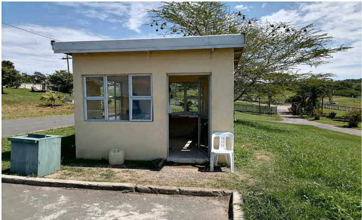
Refurbished guardhouse at the crematorium with new aluminum door and windows.
