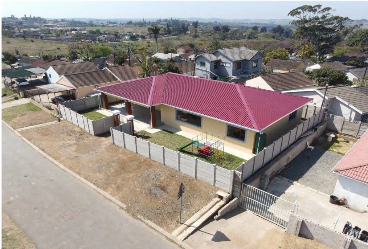
Newly constructed childcare facility in ward 28 – Shakaskraal
