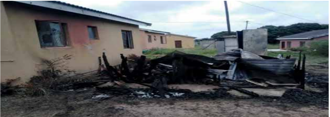
Figure 08: Conveys the aftermath following a structural fire incident in Malende Ward 9
