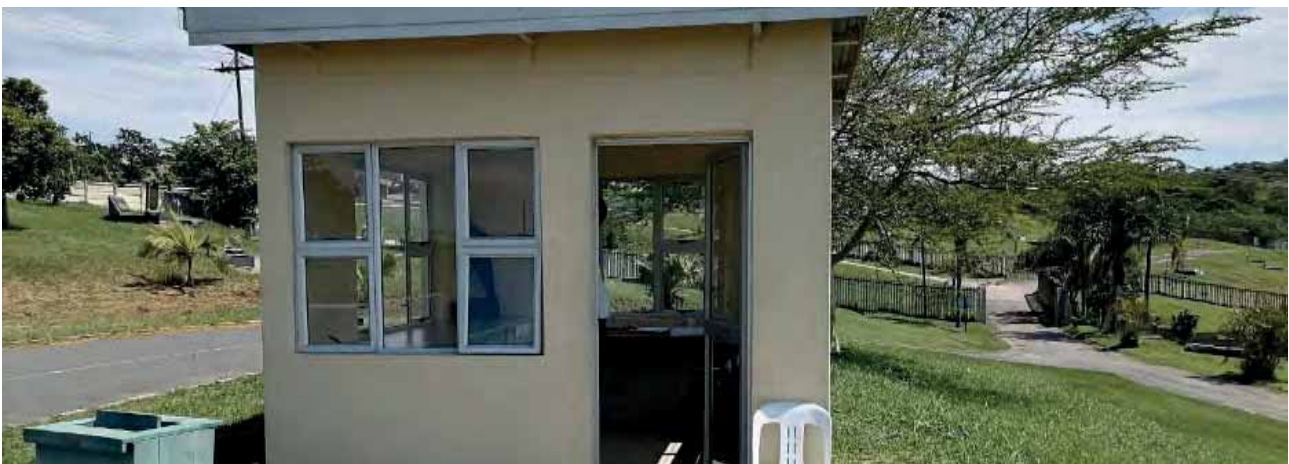
Refurbished Guardhouse at the Crematorium with New Aluminum Door and Windows.
