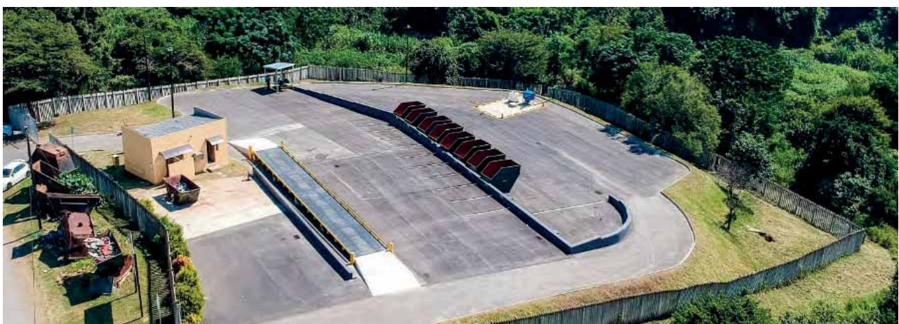
Waste Management Section - Completed KwaDukuza Waste Transfer Station
