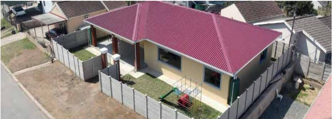
Newly Constructed Childcare Facility in Ward 28 – Shakaskraal
