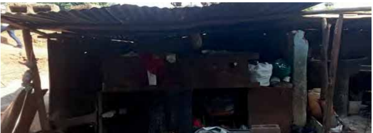
Figure 12: Conveys the aftermath following a heavy rainfall incident in Lloyd (Ward 14)
