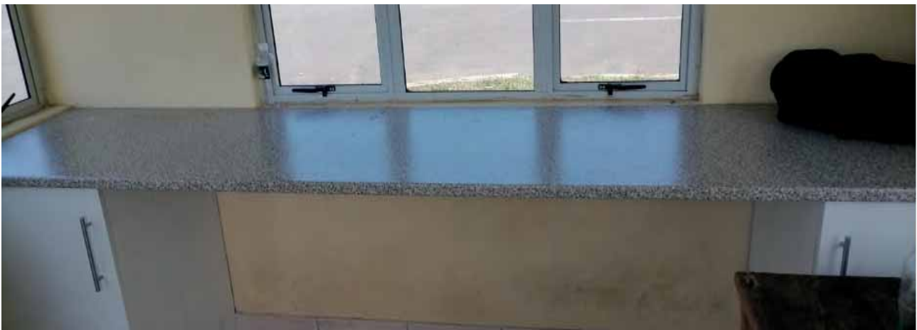
Refurbished Guard House with New Cupboards and Countertop
