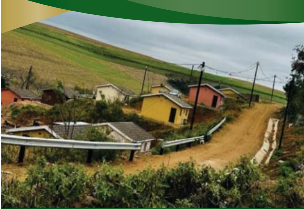
Steve Biko housing electrification completed.
