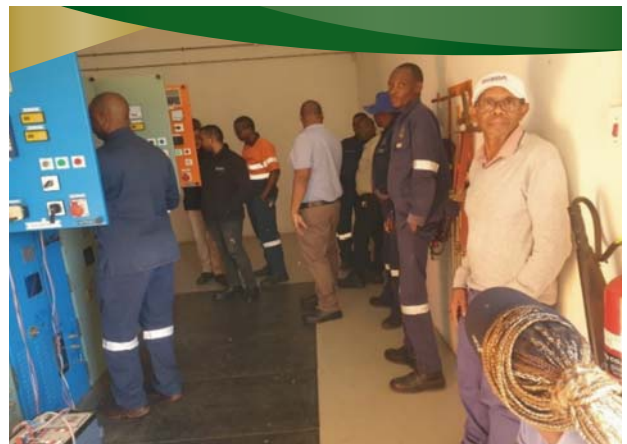
Commissioning of SCADA at Priority substation and training of municipality staff
