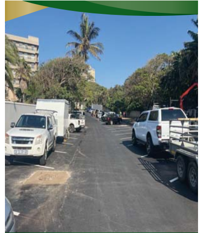
Upgrade to Willard Beach Car Park
